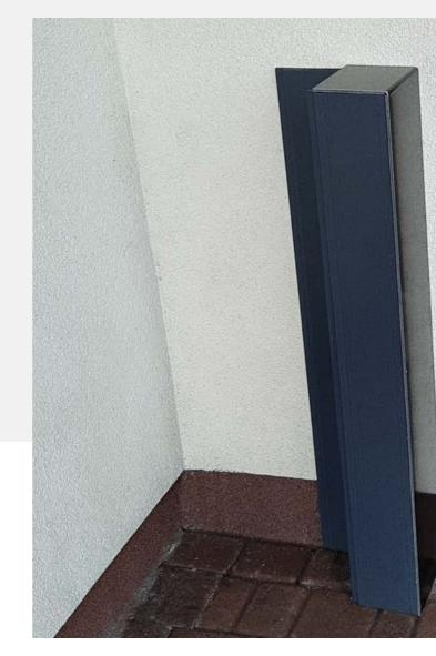
The FloodWarden barriers consist of fixed posts and adjusted to them horizontal beams assembled between the posts in emergency to form water-tight barrier. In non-emergency periods, the only visible elements of the system are the posts masked with fitting caps.
