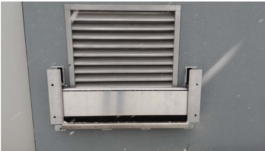
Białystok, Poland Flood protection of transformer station 0,3 m
