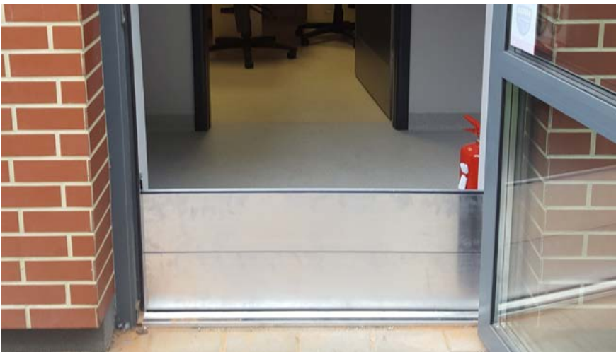
📍 Łódź 📄 Flood protection of a detached building 📏 0,4 m
