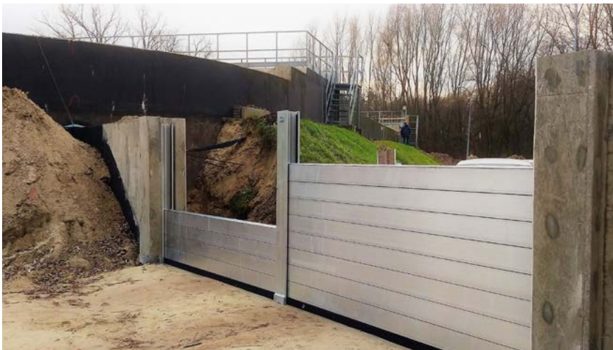
📍 Białobrzegi 📄 Mobile flood barriers in a sewage treatment plant 📏 1,65 and 1 m
