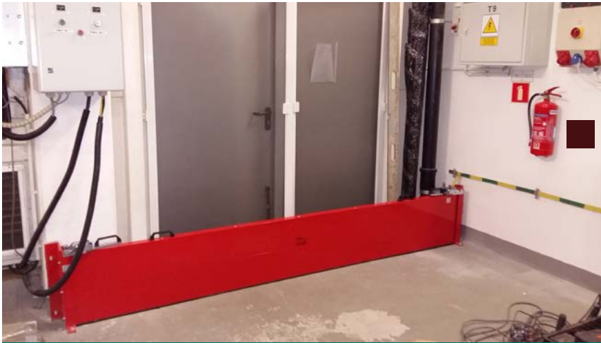
Łódź, Poland Water-tight industrial barrier. 0,4 m
