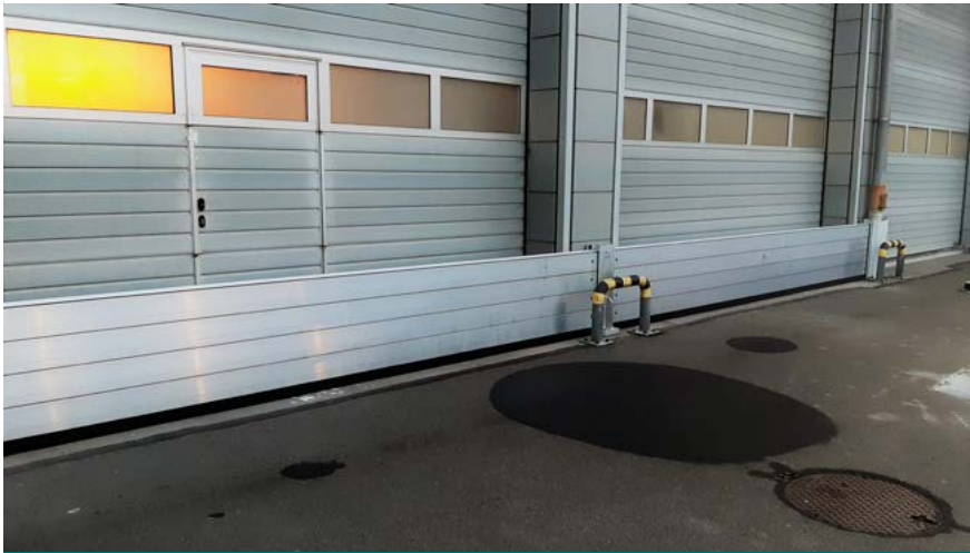
📍 Balice 📄 Flood protection of the Balice airport 📏 0,6 m
