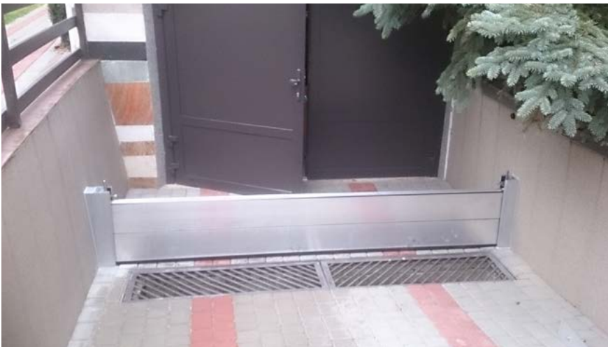
Stasiopole, Poland Flood protection of underground garage 0,3 m
