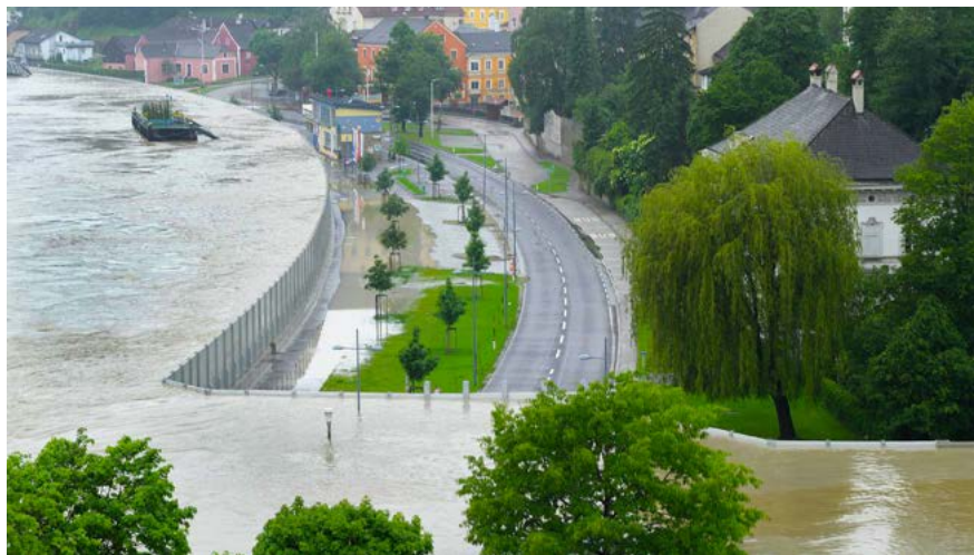
Grein, Austria Vertical flood protection system 4,6 m
