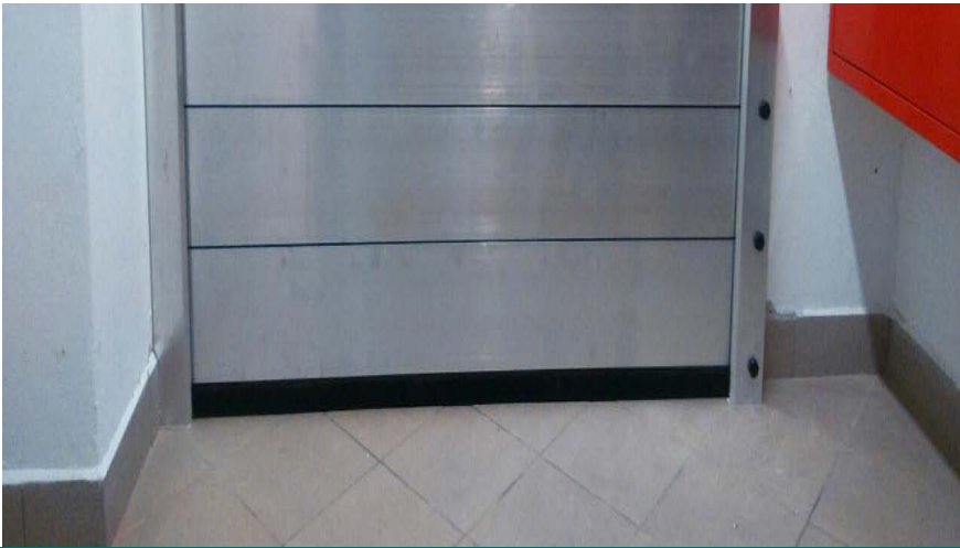
Stalowa Wola, Poland Flood protection of courthouse 0,6 m
