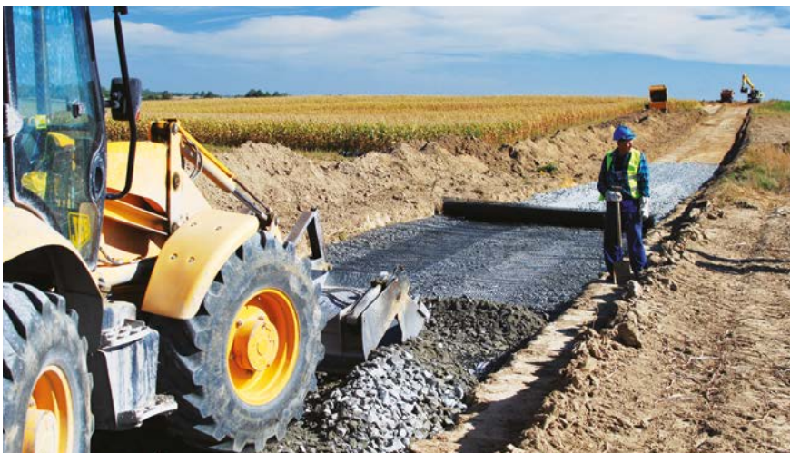
Kunów, Poland Construction of a temporary road during reconstruction of a railway track Polgrid BX 30/30 and separating non-woven fabric 7.000 m 2
