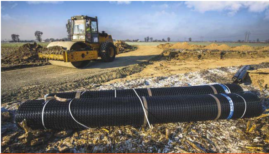
Inczew, Poland Construction of technical roads and access roads to windfarms and working platforms Polgrid 30/30 180.000 m 2
