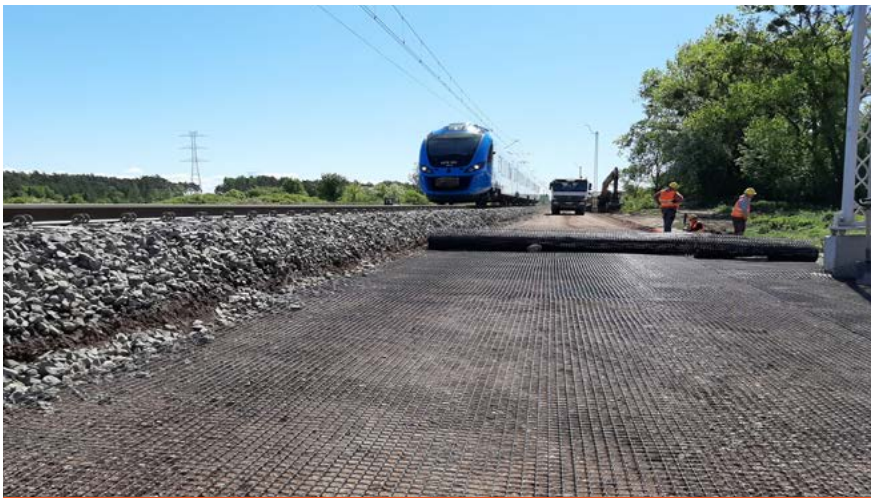
📍 Poland 📄 Geogrid used in a railway modernization project 🔲 Polgrid BX 40/40 8760 m 2
