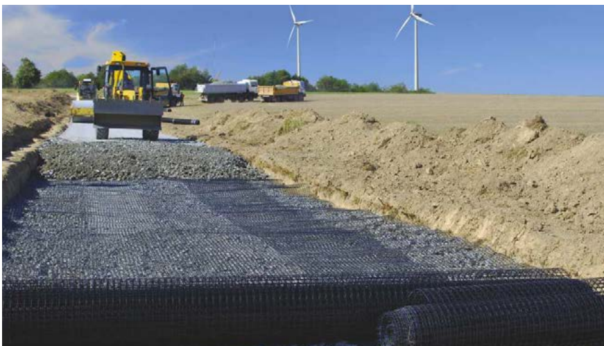
Głubczyce, Poland Construction of technical roads and access roads to windfarms Polgrid 30/30 200.000 m 2
