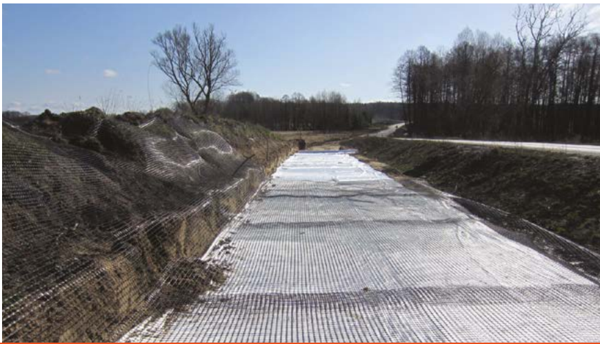
Srokowo, Poland Construction of a DW 650 road Polgrid BX 30/30 and separating non-woven fabric 30.000 m 2
