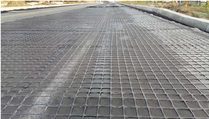
📍 Kalisz, Poland 📄 Geocomposite used to modernize and reinforce a city road 🔲 Polgrid FSR BX20/20 150PP 14.400 m 2
