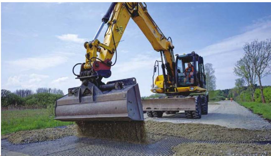
Rzepin, Poland Geosynthetic layer under a tar road Polgrid BX 20/20 and Polgrid BX 45/45 25.000 m 2
