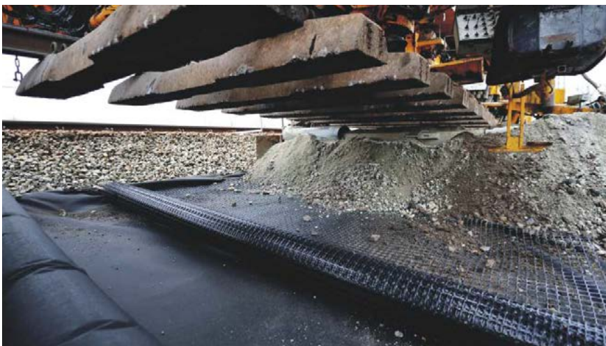
Brzezinka Średzka, Poland Reinforcement of a railway track substructure Polgrid BX 30/30 and separating non-woven fabric 7.000 m 2
