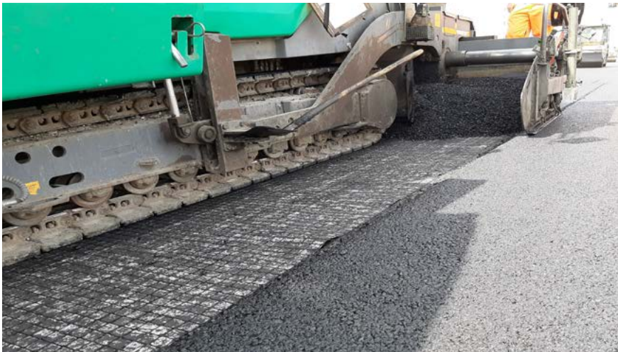
📍 Poznań, Poland 📄 The PolGrid geocomposite in a road construction project
