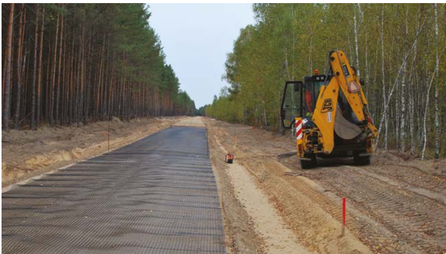
Cubin, Poland Construction of a forest road Polgrid 30/30 20.000 m 2
