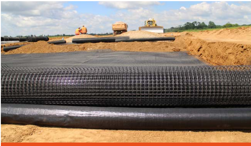
📍 Płock, Poland 📄 Construction of the ringroad around Płock 🔲 PolGrid BX30/30 82 000m 2
