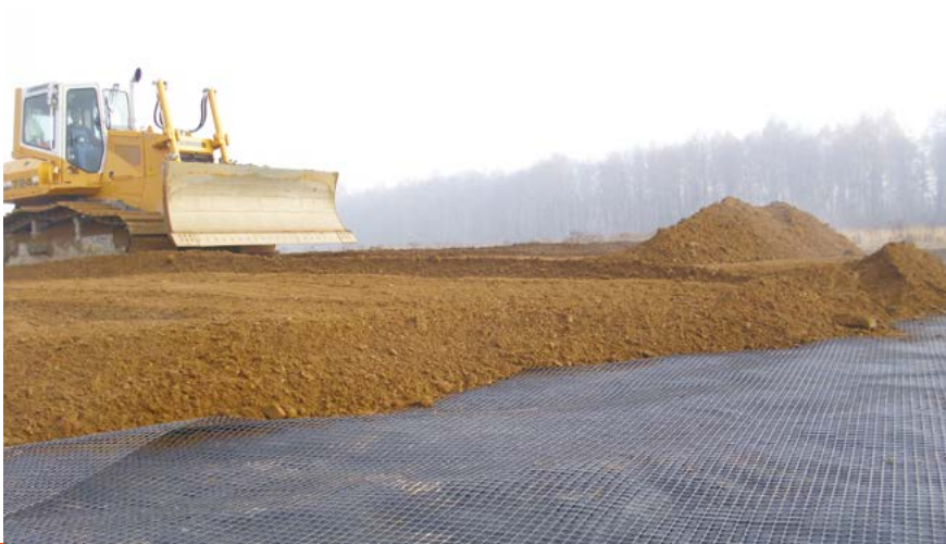
Rzeszów, Poland Reinforcement of an embankment during the construction of the S19 road Polgrid BX 20/20 and separating non-woven fabric 35.000 m 2
